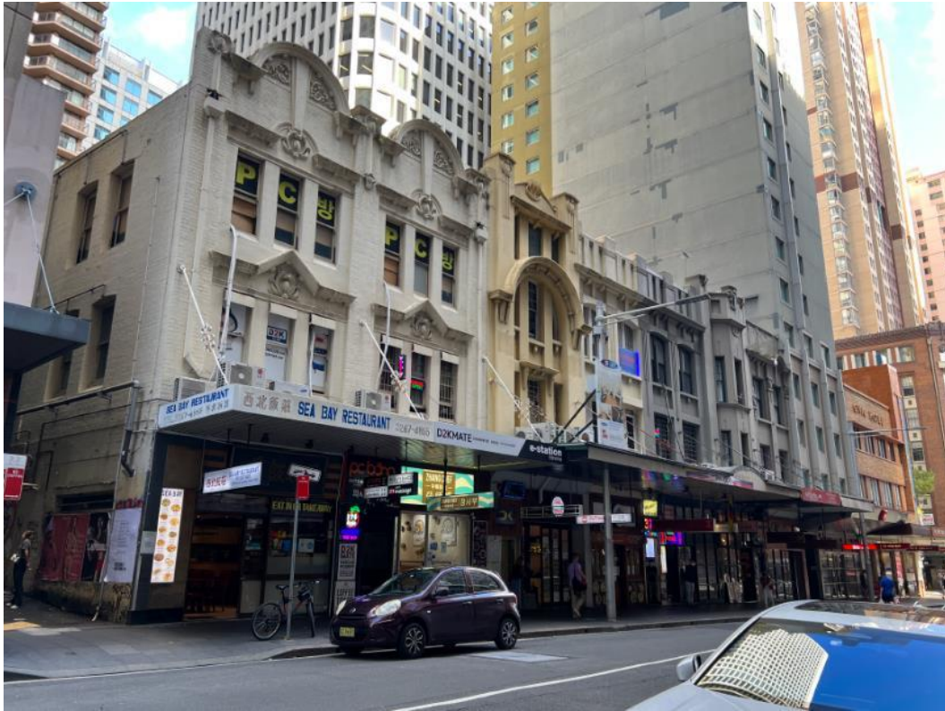
Figure 4: Subject site viewed from Pitt Street facing south-east showing existing vehicular entry to Carruthers Place
