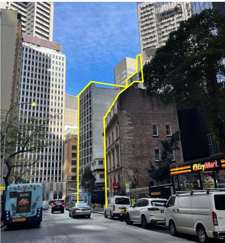
Figure 9. Eastern site, shown in yellow, viewed from Bligh Street looking south-west
