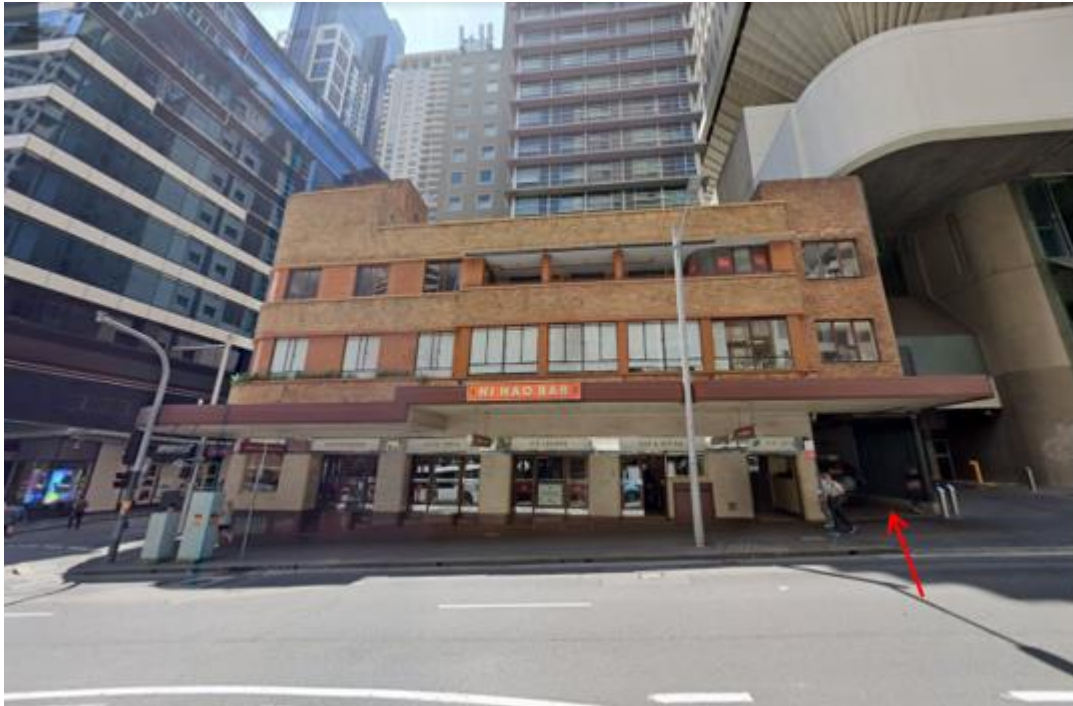
Figure 20: Goulburn Street restricted vehicular right of way marked with a red arrow
