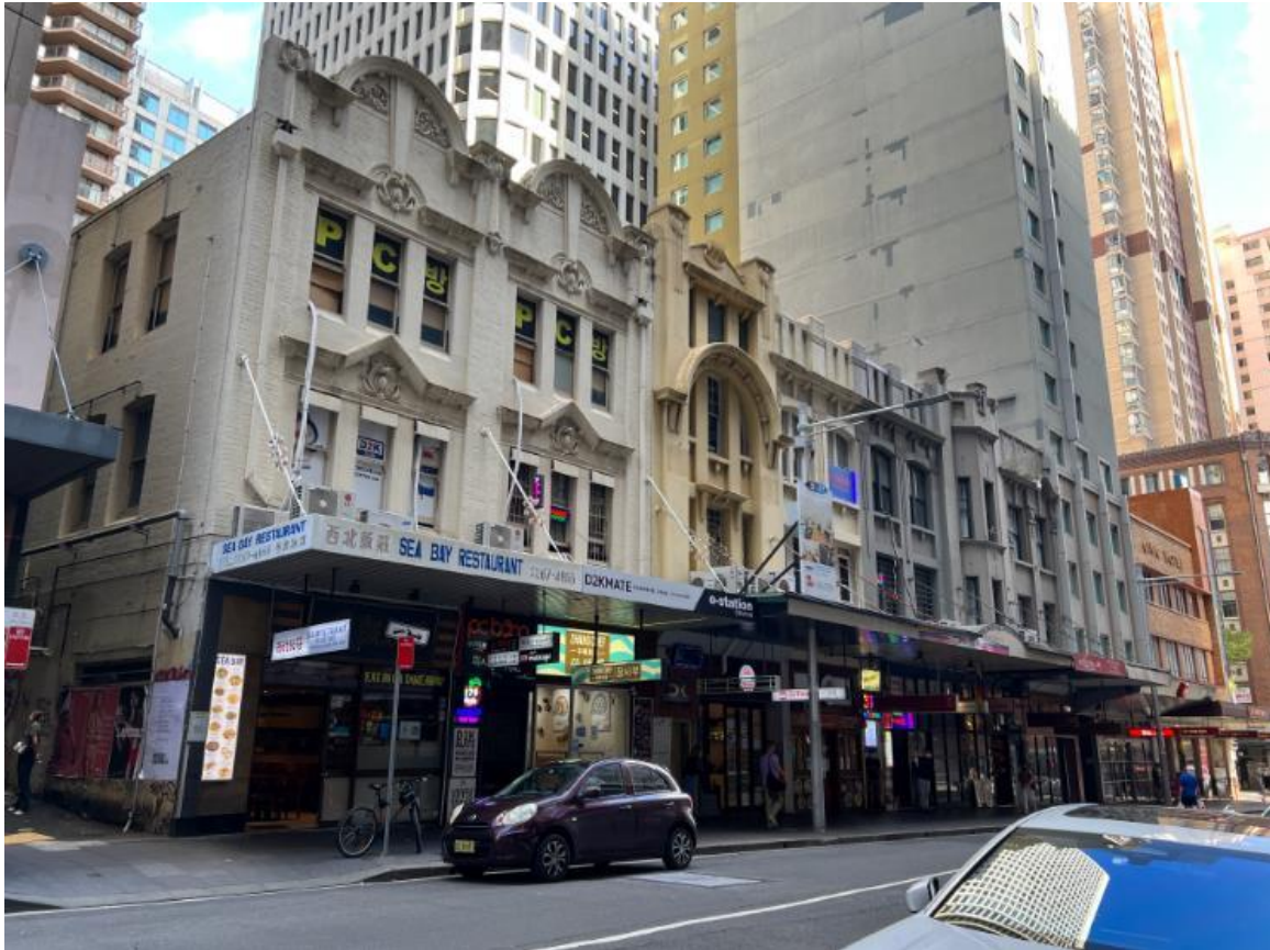
Figure 64: Present view of the subject site facing south-west
