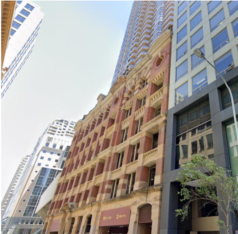
Figure 22: Museum Towers at 267-277 Castlereagh Street
